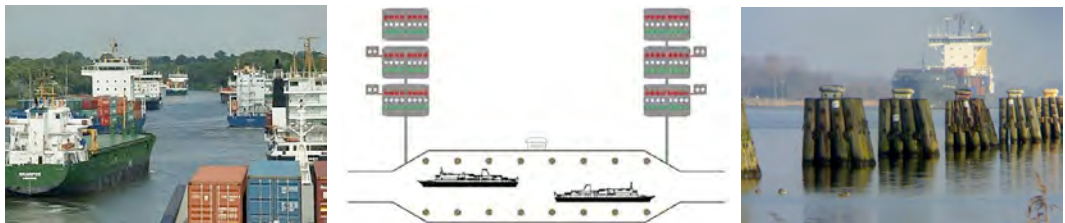
Figure 1. Glimpses of the canal and a siding with traffic lights (middle)
